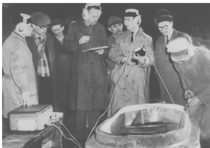
Fig. 2. Vibration measurements on the ground – Plant of “Zamech” in Elbląg. From the left: R. Ciosek, A. Czajka, Cz. Puzyna, R. Pilipkiewicz (1965).
