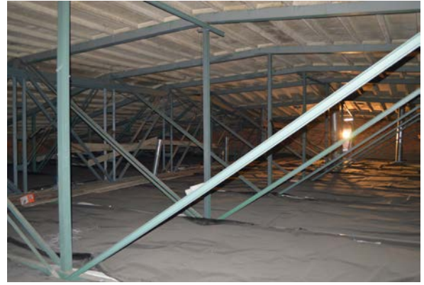
Fig. 10. Inside the ceiling of church VM.
