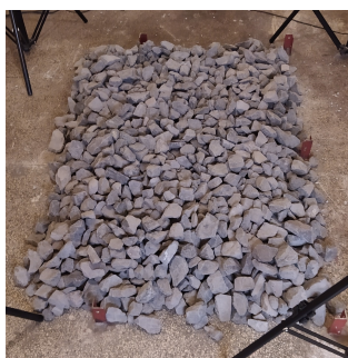
Fig. 5. Ballast layer (stone aggregate, grain size 31.5/50 mm).
