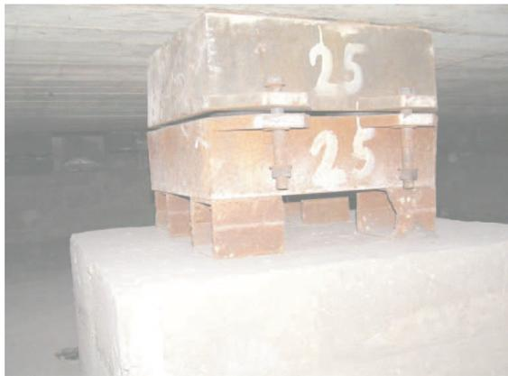
Fig. 3. The housing with springs located in the central point of support.
