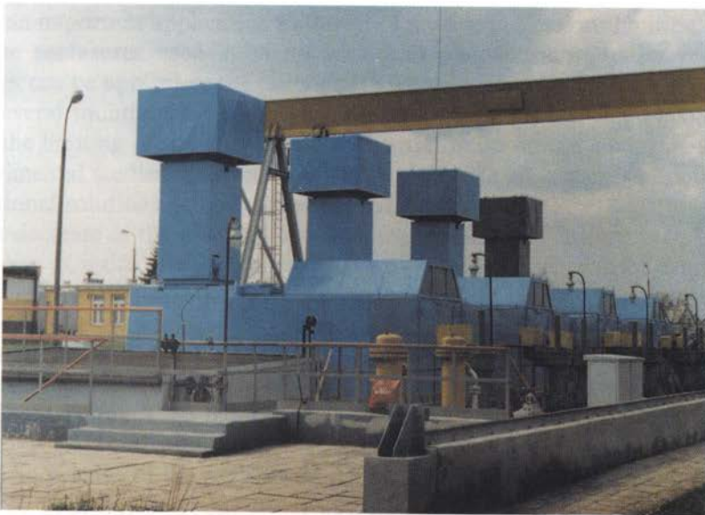
Fig. 5. Unit for partly closed enclosures (on openwork base) protecting the pumping engines in the Przepompownia Ropy ST-3 in Góry k/Płocka.
