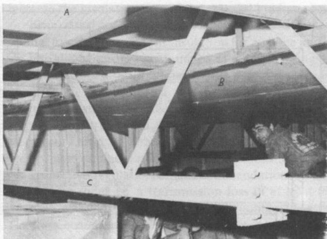
FIG. 7. View of the insulating layers gluing work
